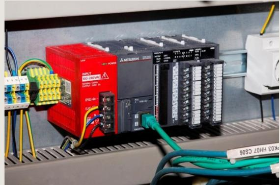
An FAG SmartController in the form of a Mitsubishi Electric PLC from the MELSEC L-series operates as a bidirectional gateway between the customer controller and sensors in the condition monitoring system. [Source: Mitsubishi Electric Europe B.V.]
