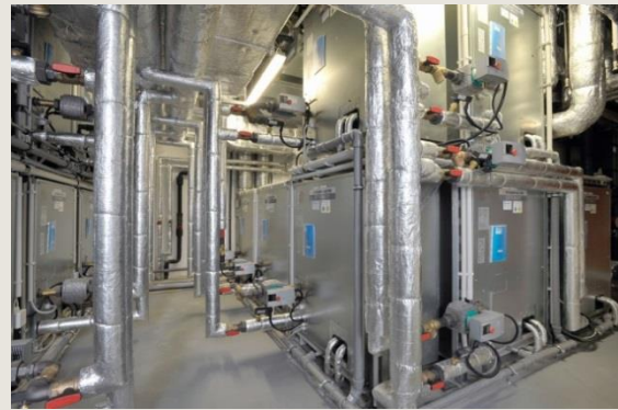
There are 17 City Multi Series outdoor units in the technical center.
